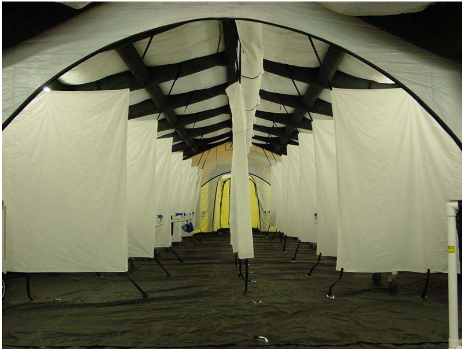
Patient Privacy Curtains and Center Divider installed in Mdl 860
